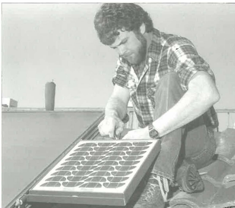
Andy Pesce working on PV pump for solar water heating (February 1988)
