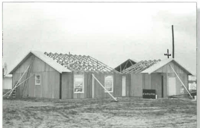
PV house under construction (January 1980)
