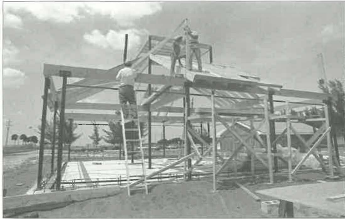
Passive Cooling Lab under construction (June 1981)
