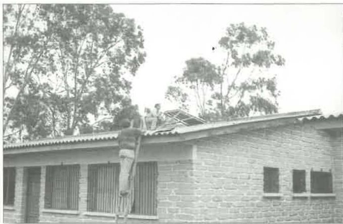
South American Health Clinics PV Project (July 1986)
