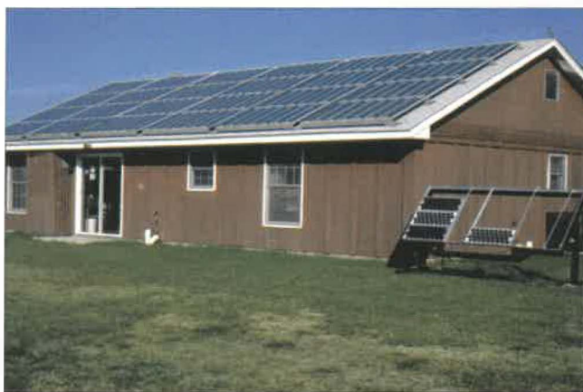
PV house with 5-kw of PV
