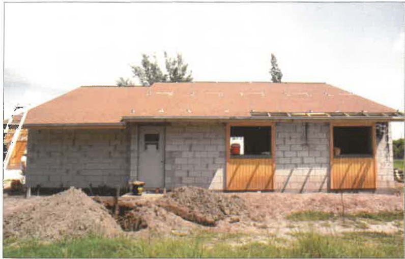
SE RES Prototype house under construction (March 1983)
