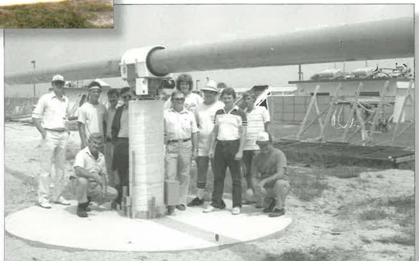
Solar trackers – Joe Harris and crew (July 1984)
