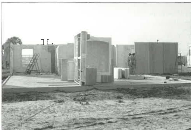
PV house under construction (January 1980)
