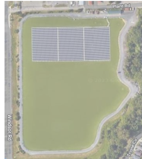
Windsor, CA 1.78 MW, Water Treatment, Surface covered 22%
