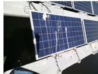
From a floating solar PV in FL: Bird dropping completely blocked a PV cell, and, the cell is operating at 138°C.
