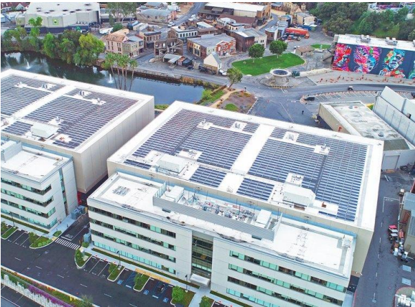
Universal Studio Lot Installs 1.5 MW of Solar on Stages
