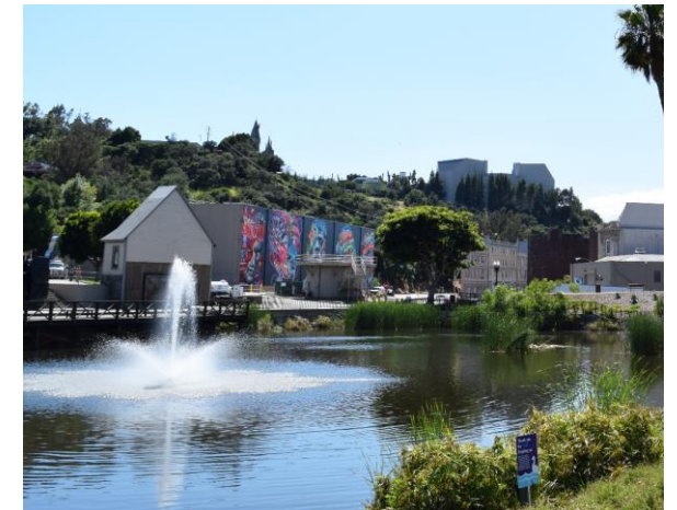
Studio Lot Irrigates with Recycled Water & Treats Stormwater On-Site
