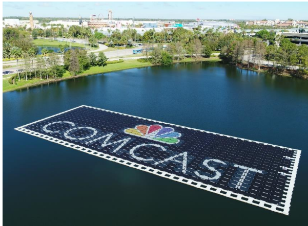
Universal Studios Orlando Builds Floating Solar Array
