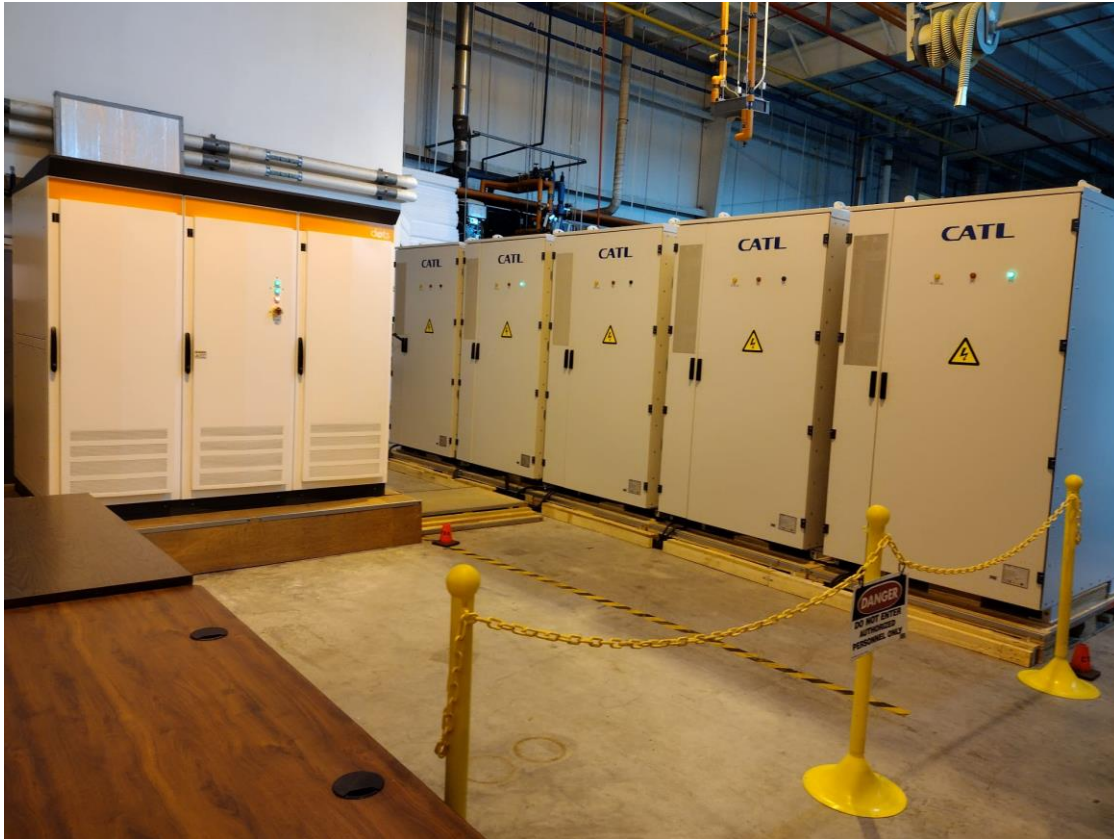
Research & Development Lab at FSEC in Central Florida.
