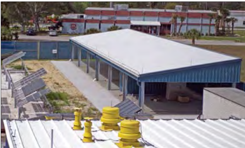
FSEC's distributed generation test facility (March 2004)
