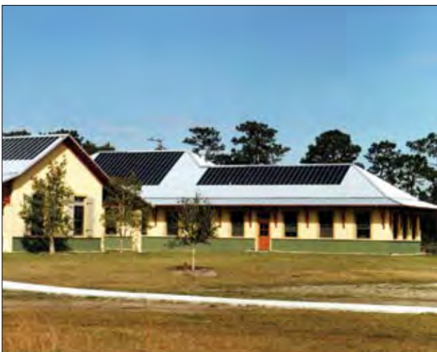
Roof integrated PV on Florida Nature Conservancy, Kissimmee, FL (January 2000)
