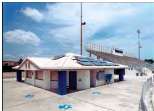
PV at Dr. Phillips High School, Orlando, FL (April 2002)
