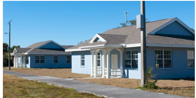
FSEC researches a variety of energy system improvements to homes in a hot-humid climate using, two onsite, heavily-instrumented and identical side-by-side homes with simulated occupancy.
