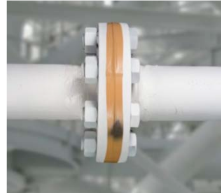
A hydrogen detection safety tape developed at FSEC, in partnership with NASA, provides a visual indication when hydrogen (odorless and colorless) is leaking.
