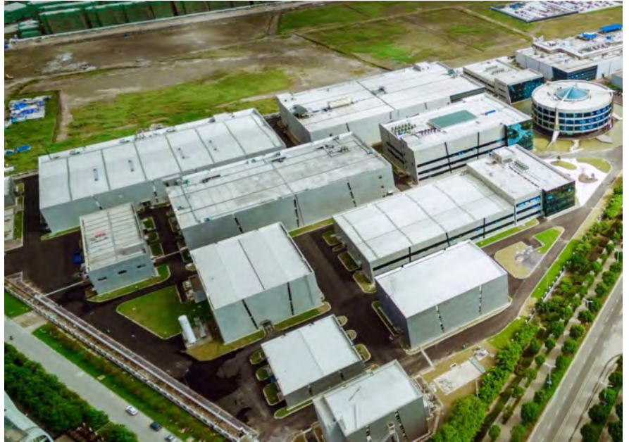
Microvast manufacturing facility (Phase I and II), Huzhou, Zhejiang, China.
