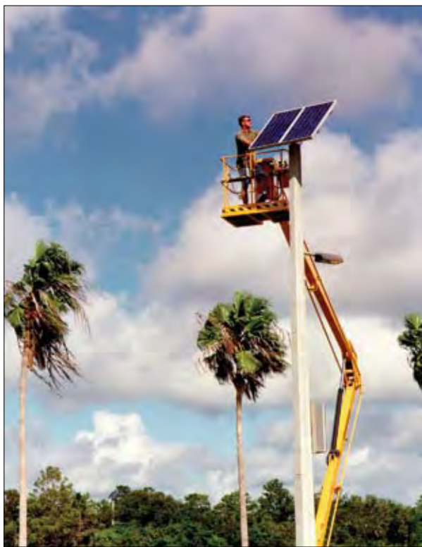
Donard Metzger installs PV light system
