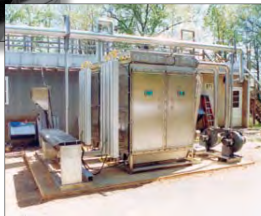
Full-scale 650-SCFM detox reactor installed at Naval Surface Warfare Center, Indian Head, MD (October 1998)
