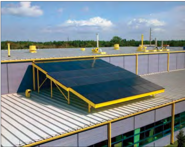
12-kWp PV array on low bay roof (January 1997)
