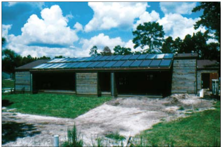
HUD residential solar air-conditioning demonstration project (1977)
