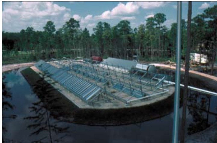
I-95 Welcome Station Solar Air Conditioning Project, under construction (1978)
