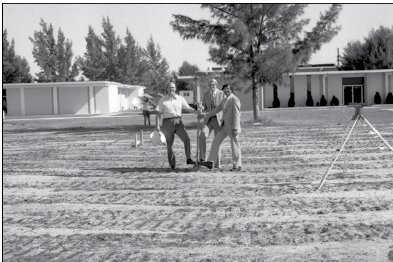
PV house site ground breaking -- Leroy Nash, David Block, Subrato Chandra (January 1980)
