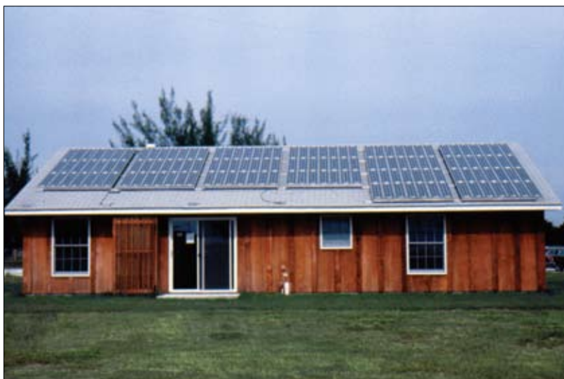
Partially completed FSEC PV house (1980)
