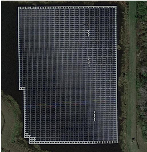
Altamonte Springs, FL 960 kW, Storm Water Pond, DC/AC 1.16
