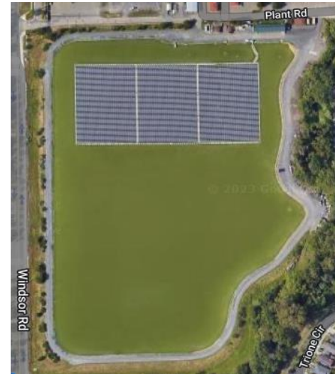
Windsor, CA 1.78 MW, Water Treatment, Surface covered 22%
