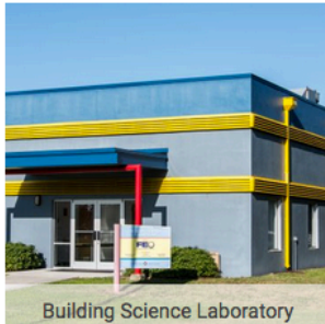
Building Science Laboratory
