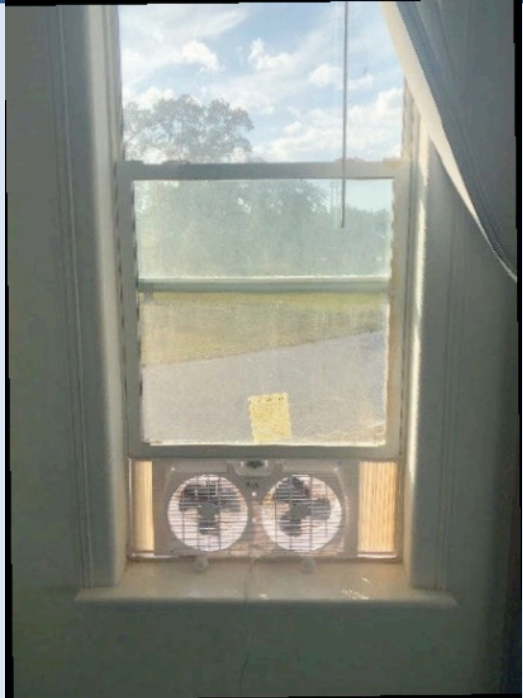
a. An inexpensive window fan can aid with containment
