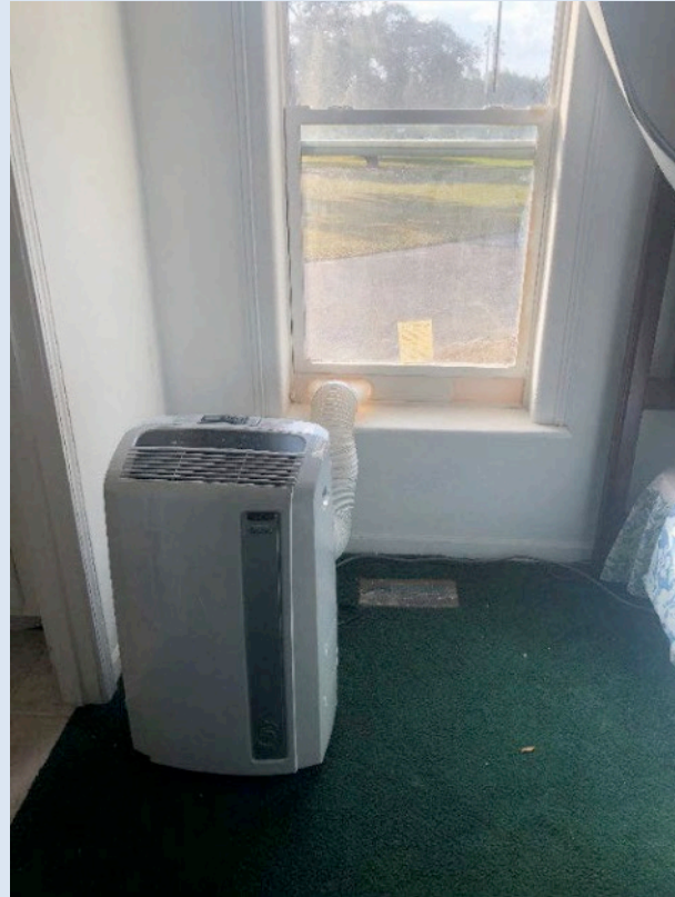
b. Portable air conditioner can be used to aid with containment, and provide comfort to the isolation zone.
