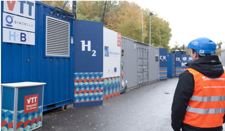
Plug Power Electrolyzers: Hydrogen from electrolysis combined with CO 2 captured from air/industrial sources to produce Biomethane & Biofuels
